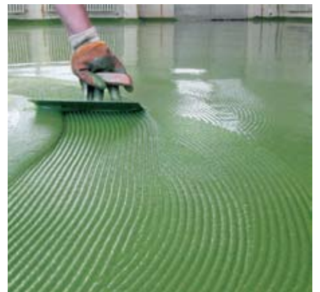
Application steps of EPOLIT ANTISTATIK (MB Namenska Lučani, 1500 m 2 )
